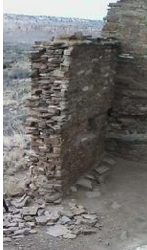
Chaco Core and Veneer Construction, Tsin Kletzin Left and Hungo Pavi Right At Aztec North the Core Stones are Replaced by an Adobe Mass
