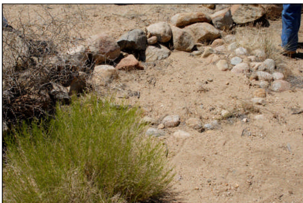
Goat Hill Check Dam with Spill Pool
