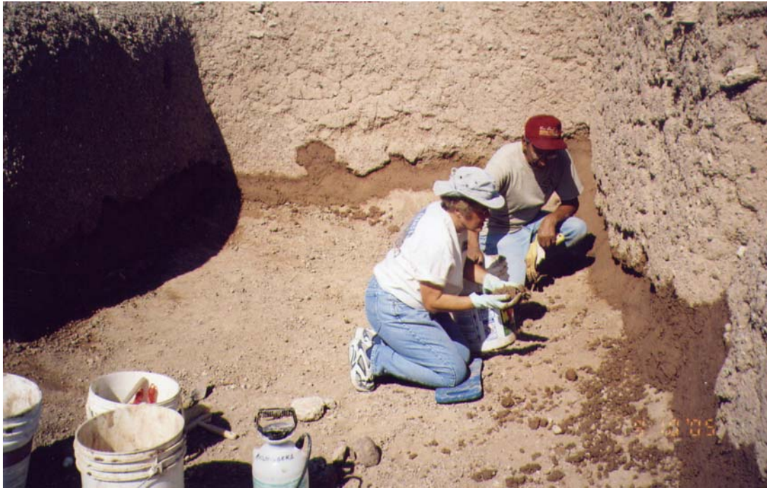
Walt Lesko & Donna Beng repairing local erosion with Soil Shield-Ls amended mud.
